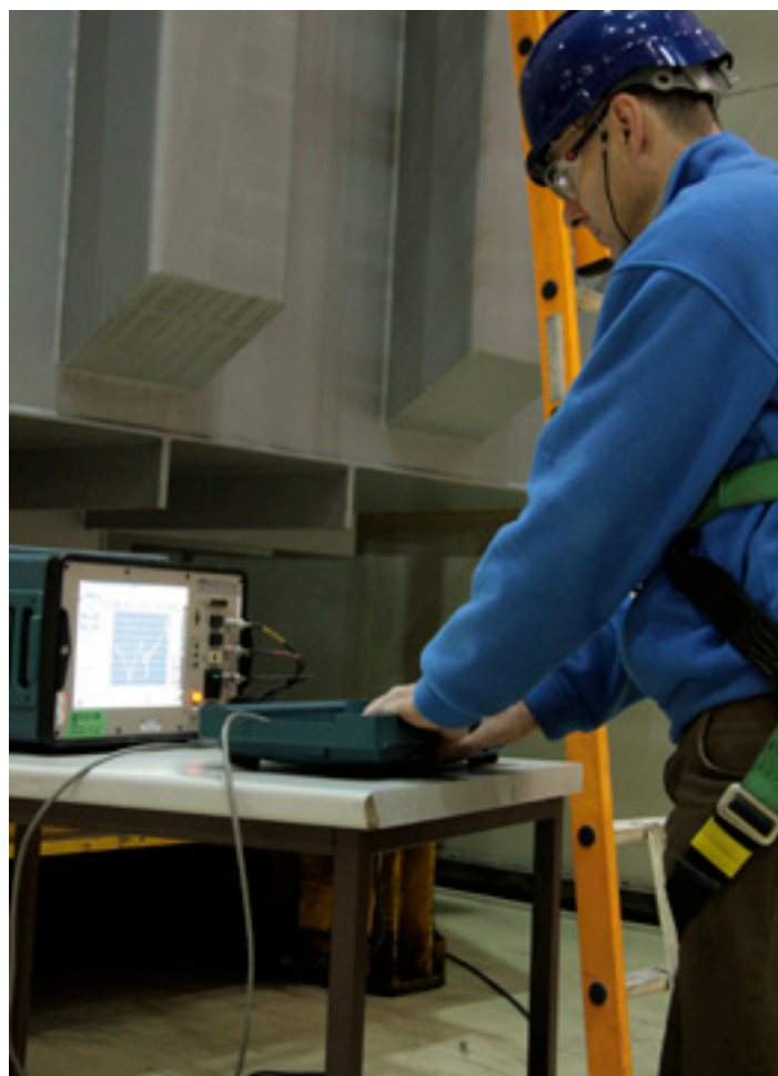
Each transformer is SFRA fingerprinted in the test bay >
